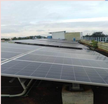
12KW Solar Power Panels
